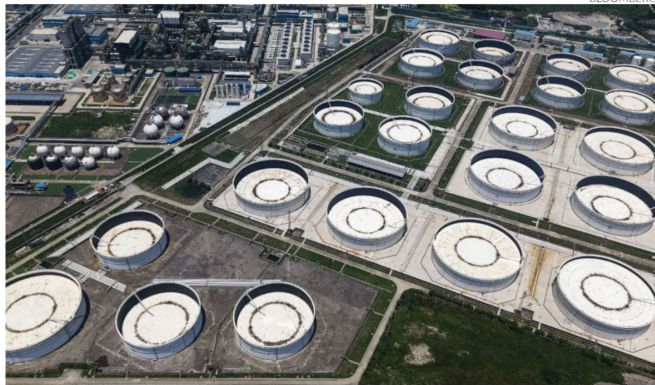
Oil storage tanks at a refinery in China. China's stockpile of crude oil is enough to help her cushion the effects of the conflict in the Middle East for the moment.
